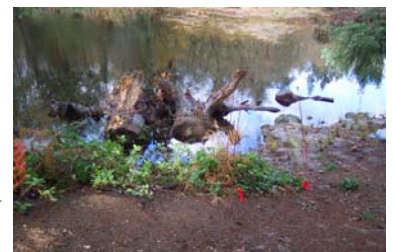
Soft armoring with large woody debris at Crescent Creek
